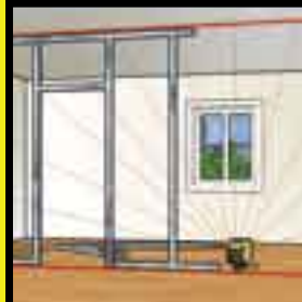
VERTICAL LEVELLING & SQUARING
