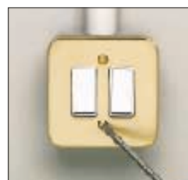
6 Fix face plate onto grid.
