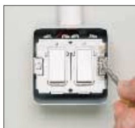
5 Fix wired switch/grid assembly into box.
