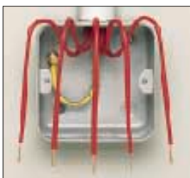
1 Install box and enter cables.
