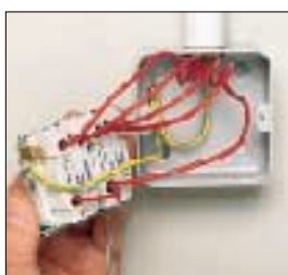
4 Connect wires to relevant switches & earth terminals.
