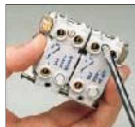
3 Fix switches into grid.
