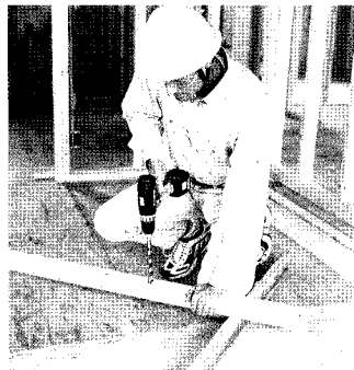
Drilling into wood
