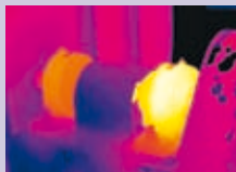
Overheating bearing cap
