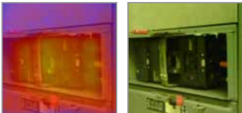
Normal operating temperature on mission critical breaker
