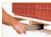
PLACE AROUND THE FIRST TWO-WAY STRINGER
