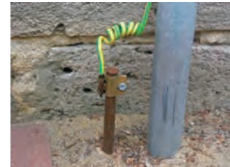
A typical earthing electrode (left of gray pipe), consisting of a conductive rod driven into the ground.
