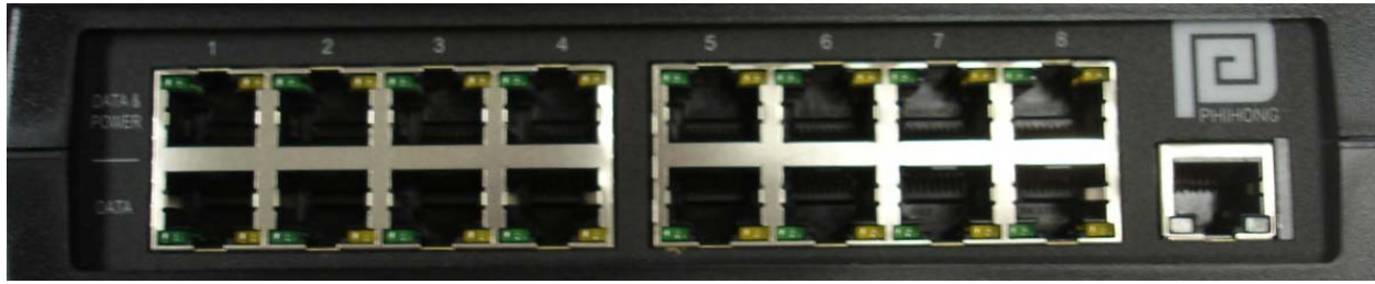
Fig 1 Front side of Midspan
