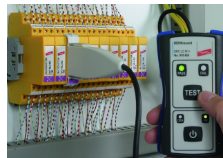
Snap-on LifeCheck sensor
