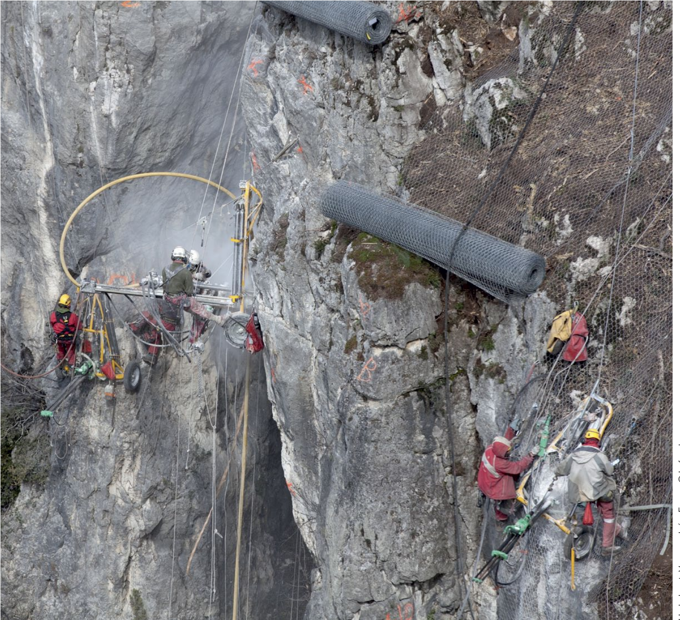
Hydrokarst, Voreppe, Isère France © Lafouche
